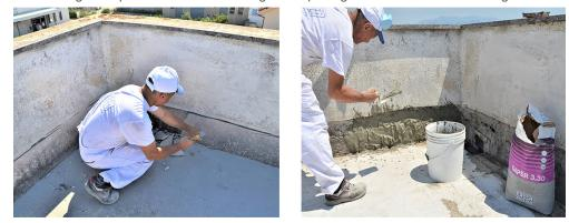
The AQUAZIP ELASTOBAND will be positioned along the connections between the horizontal plane and the vertical overlaps. The strip must be laid continuously on the application surfaces, first applying an at least 2 mm thick layer of AQUAZIP ONE waterproofing membrane, to a width exceeding the strip and making sure to leave the centre part free. For perfect sealing of the corners, use the appropriate preformed elements.
