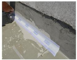
The AQUAZIP ONE waterproofing system will also be applied on the vertical overlaps, and after suitable curing will be covered with a coat of KI7 or KZ 35, lime and cement base coat plasters/renders for exteriors and interiors, mixed with a solution of water and AG 15 (1 part AG 15 to 3 parts water). The base coat plaster must be fine-float finished, embedding wide-weave synthetic plaster reinforcing mesh during application.
