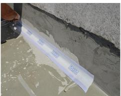
The AQUAZIP fast waterproofing system will also be applied on the vertical overlaps, and after suitable curing will be covered with a coat of KI7 or KZ 35, lime and cement base coat plasters/renders for exteriors and interiors, mixed with a solution of water and AG 15 (1 part AG 15 to 3 parts water), dispersion of synthetic resins for cement-based products. The base coat plaster must be fine-float finished, embedding wide-weave synthetic plaster reinforcing mesh during application.
