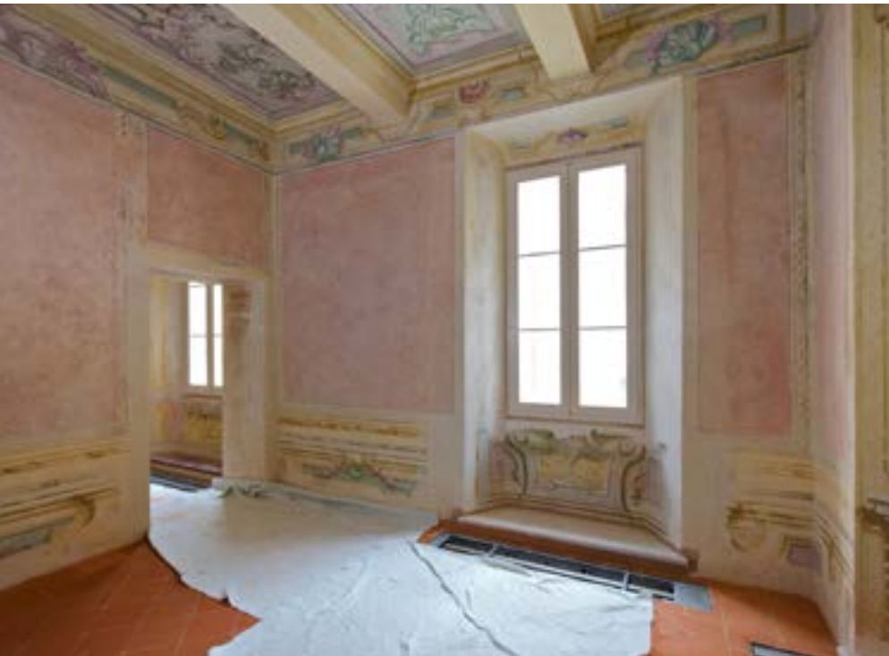
Restoration of wall decorations
