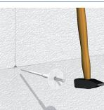
The anchors are inserted at each joint and, if the adhesive bond needs to be reinforced, a further one or two are applied in the centre (there must never be less than 5 anchors per sq.m).
